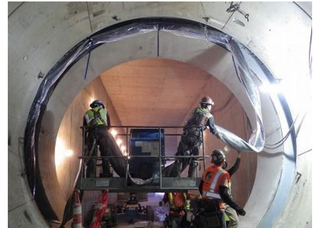
6. Temporary setting of \Omega seal
