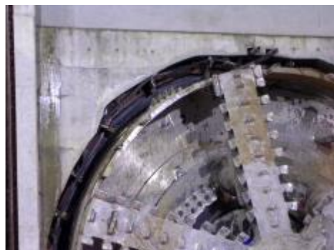
Situation of pre-cutting bit just after bulkhead had dismantled
