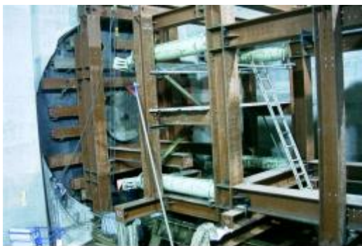
Installing movable bulkhead and back anchor
