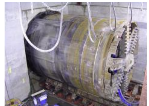
Completion of TBM arriving
